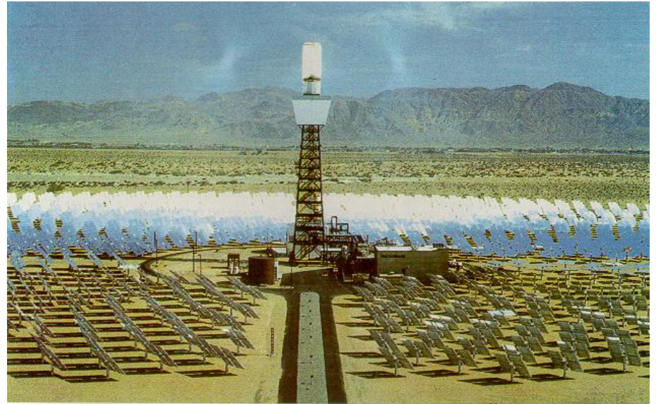
Fig. 1.6 Solar-1 pilot plant (10 MW e ) under test in Barstow, Calif. (U.S.A.)
